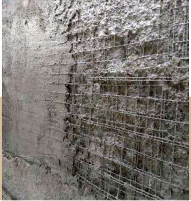
**STUCANET SN** is a high galvanized or stainless steel electro-welded mesh, suitable for the restoration of masonry structures (brick, stone, tuff, etc.) as are MX-RW High Performances and MX-CP Lime mortars. When properly applied to the substrate, it gives the plaster suitable resistance to the stresses to which the underlying masonry is subject.
