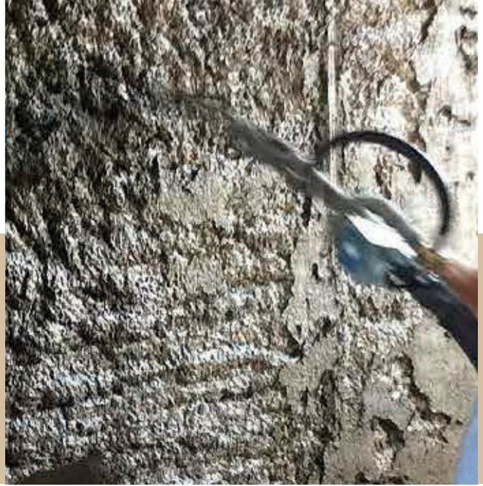
**MX-RW High Performances** is a premixed mortar based on a high pozzolan hydraulic binder and low salt content, select aggregates, additives, and polypropylene fibers.
