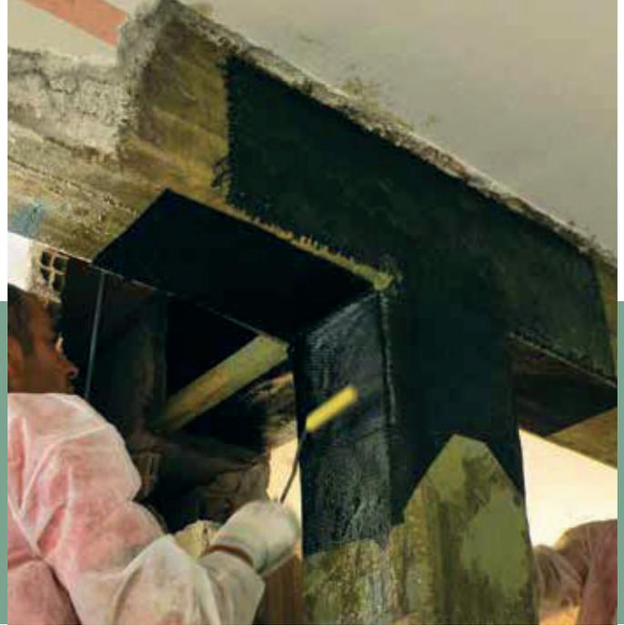
**C-QUADRIWRAP** is a four-axis carbon fiber connection system for the construction of FRP structural strengthening systems.
